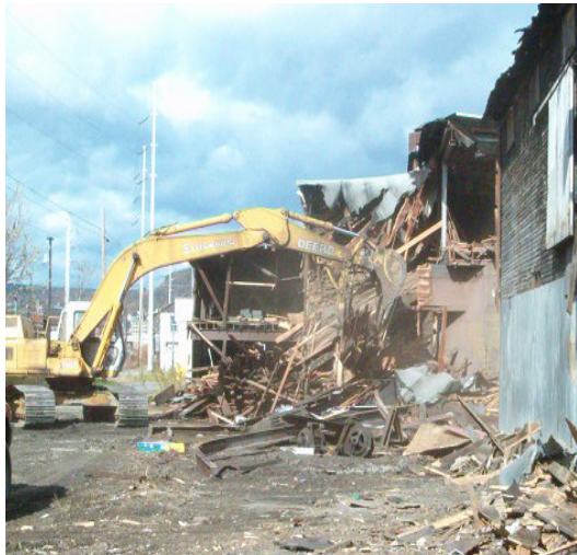
Above: Demolition and clean-up of the former Johnstown Planing Mill.
