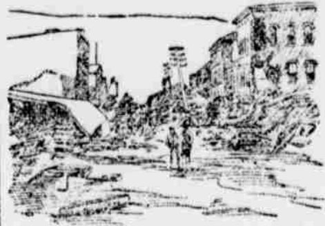
CORNER MAIN AND CLINTON STREETS. (Rains of Harbort House on Right.)
